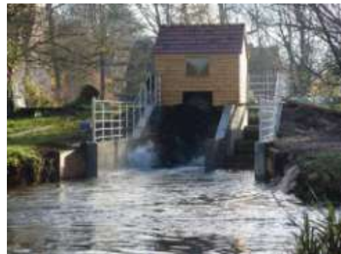
Bindon Mill hydro electric
