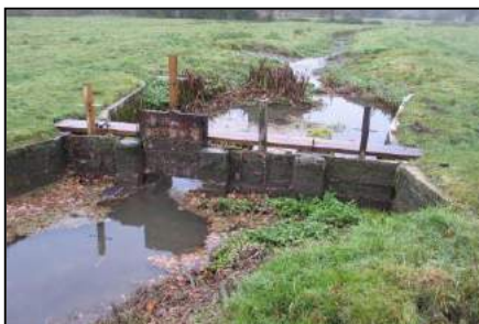
Restoring hatches in Lower Woodford
